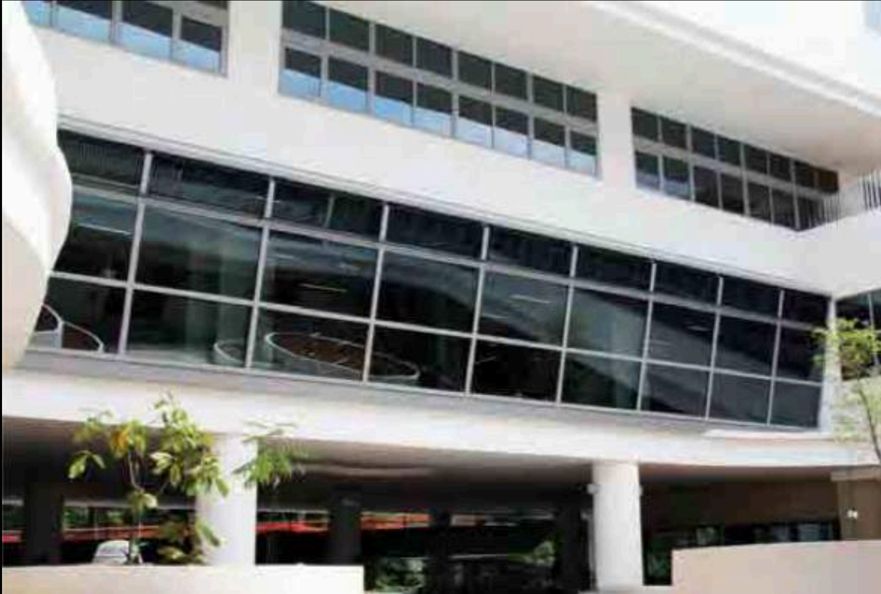
UCWSEA pilot installation, Singapore, 2015
